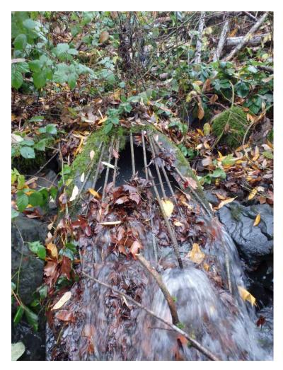
Photo 9 24-inch Outfall from energy dissipation Concrete Box at outfall from 36-inch Pipe
