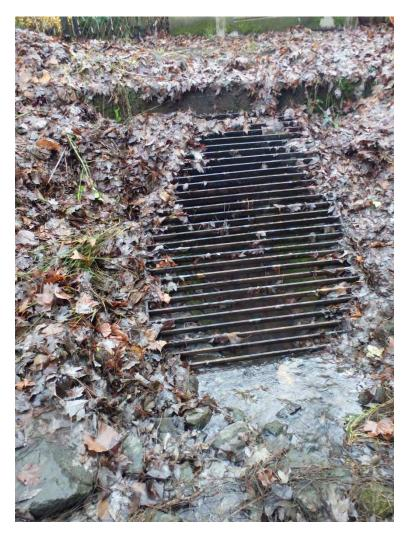
Photo 7 36-inch culvert under SW Willow Creek Drive
