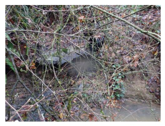
Photo 16 Perched Culvert on Right Bank
