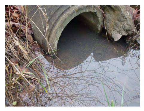
Photo 3 Downstream of culvert with gravel accumulation
