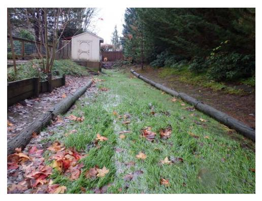
Photo 5 Vegetated channel with taller banks and logs channeling flow
