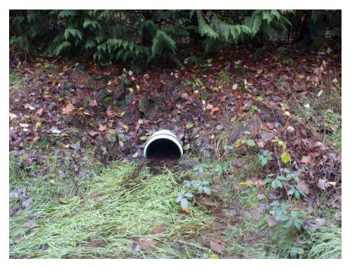
Photo 6 Partly submerged 18-inch CCP contributing culvert
