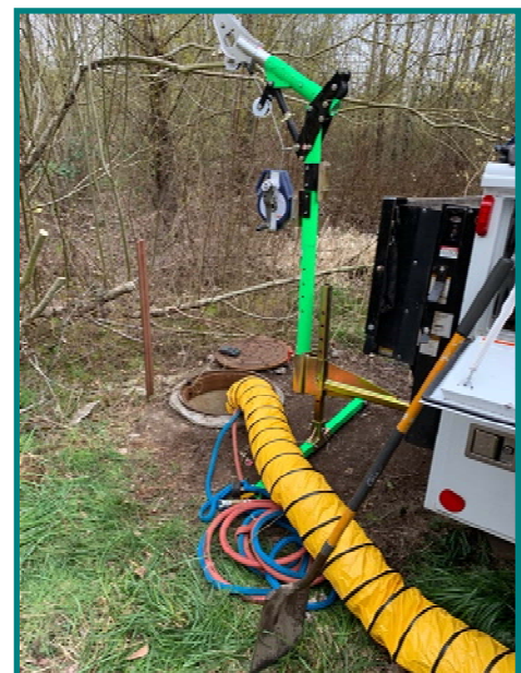
Equipment boom aids in accessing manhole
