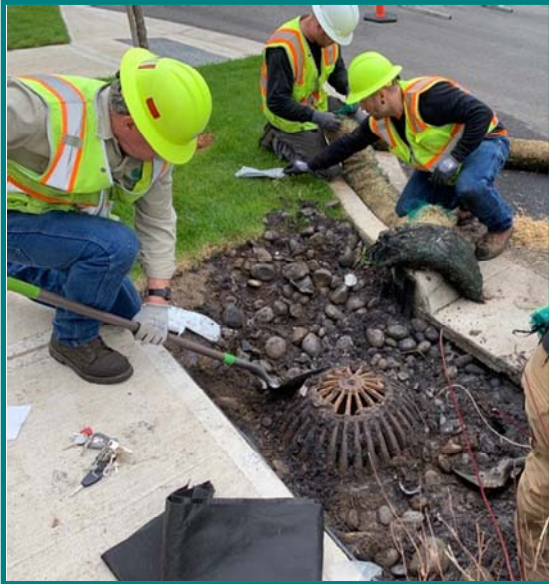
Staff cleaning a stormwater inlet and installing BMP devices
