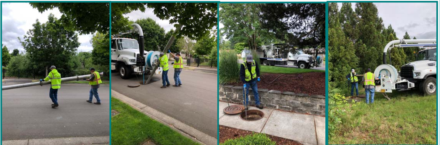
Paul H. and Paul W. inspecting and cleaning sanitary system
