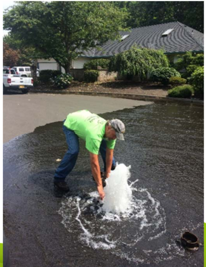
Water Technician Chris Reece opens a blow off valve on Ironwood Court in Charbonneau.
