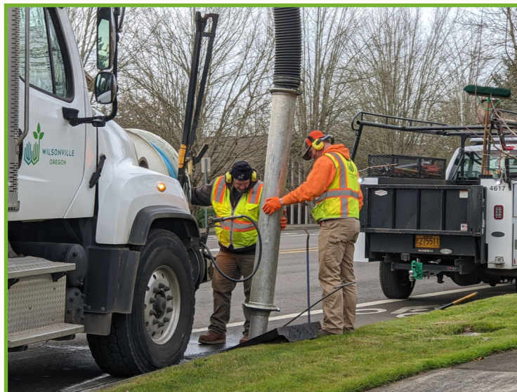
Cleaning an inlet with the vacuum truck
