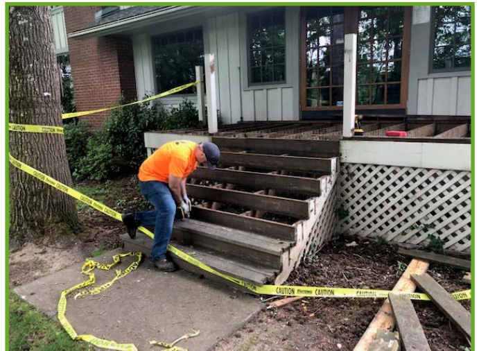
Removing stair treads
