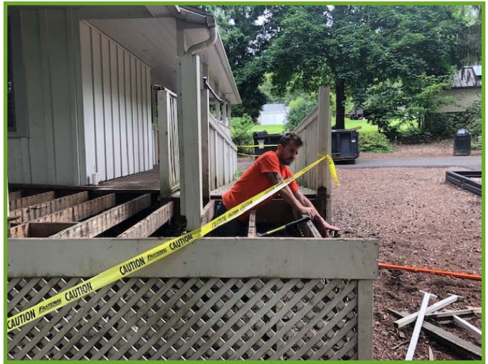
Removing floor decking
