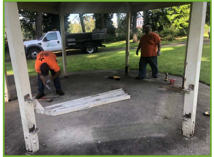
Removing the side posts from the Gazebo
