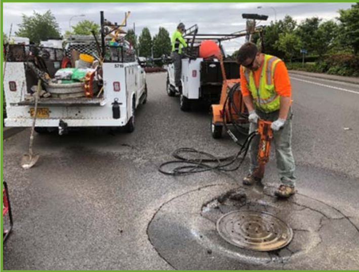
Staff digging out the asphalt and manhole riser ring
