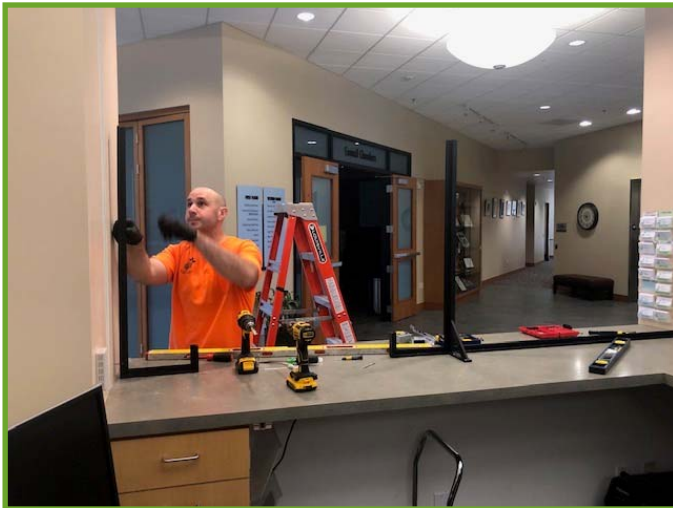
Installation of sneeze guard at City Hall front counter
