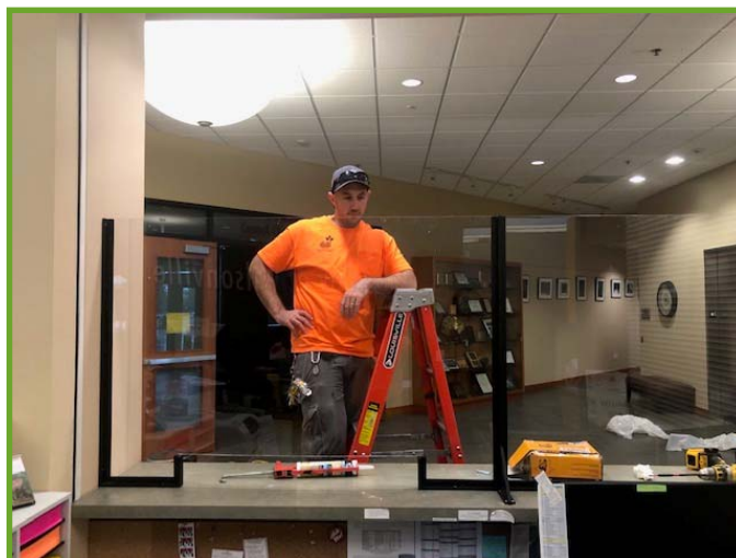
Double checking the completed guard installation
