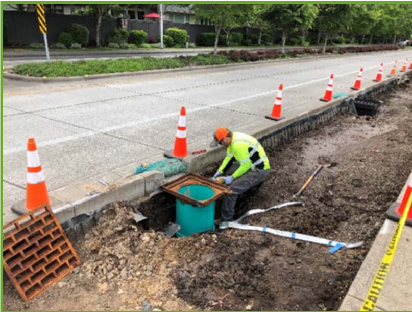
Installation of catch basin
