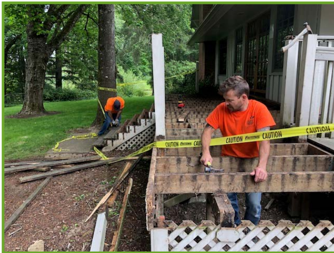
Checking the integrity of the floor joists
