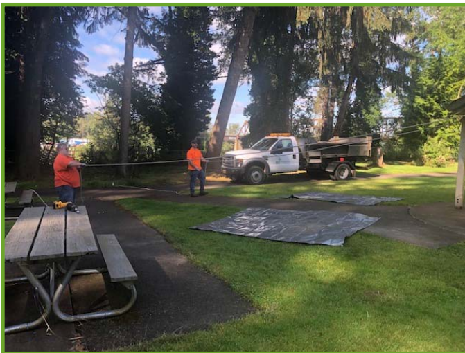
Carefully pulling down the Gazebo
