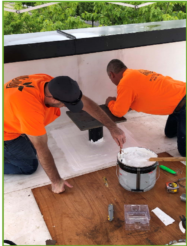
Installation of waterproofing around the Davit Arm mounting bracket
