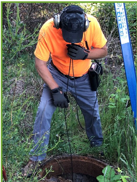
Listening for a leak
