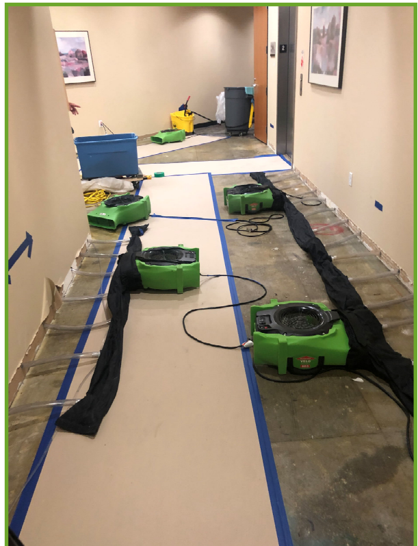
Drying the lobby —the elevator stayed dry!
