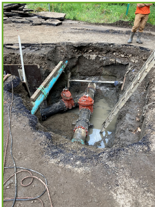
Temporary diversion of wastewater
