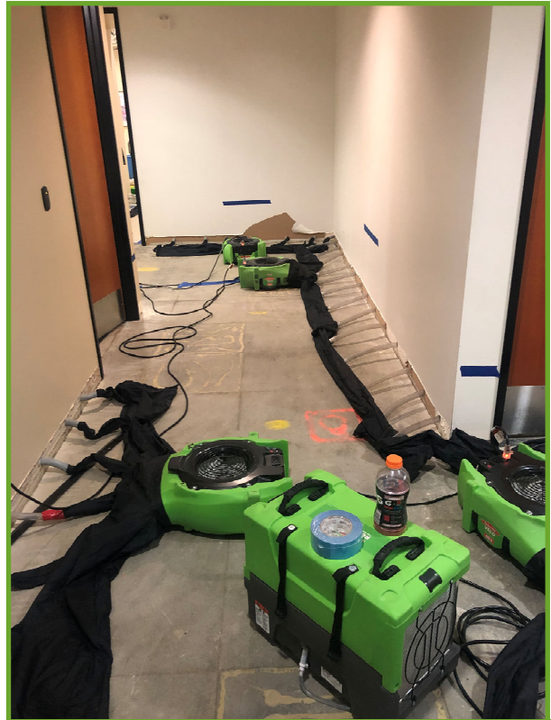
Drying the hallways outside the restroom
