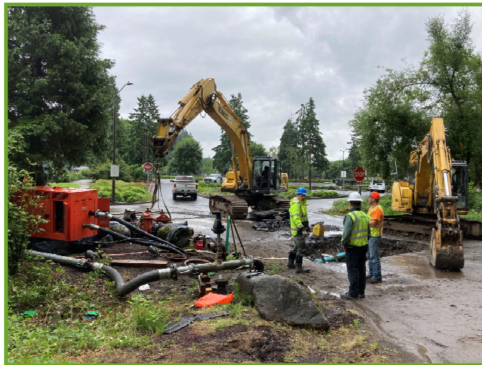
Excavating the old force main pipe
