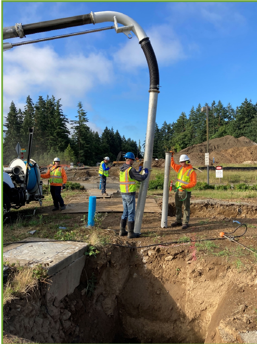
Potholing to find the water line
