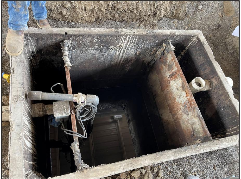
Oil separator vault—bad, removed from service
