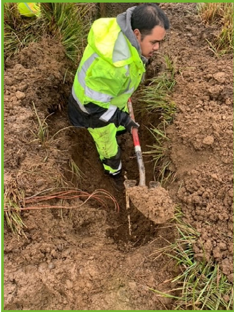
Digging around a line
