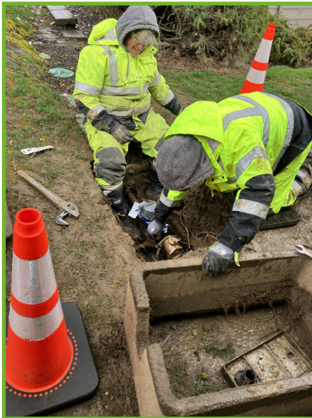
Angle stop repair
