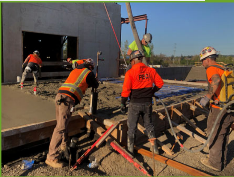
Pouring the slab on grade concrete
