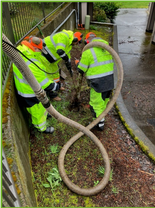
Digging around the site
