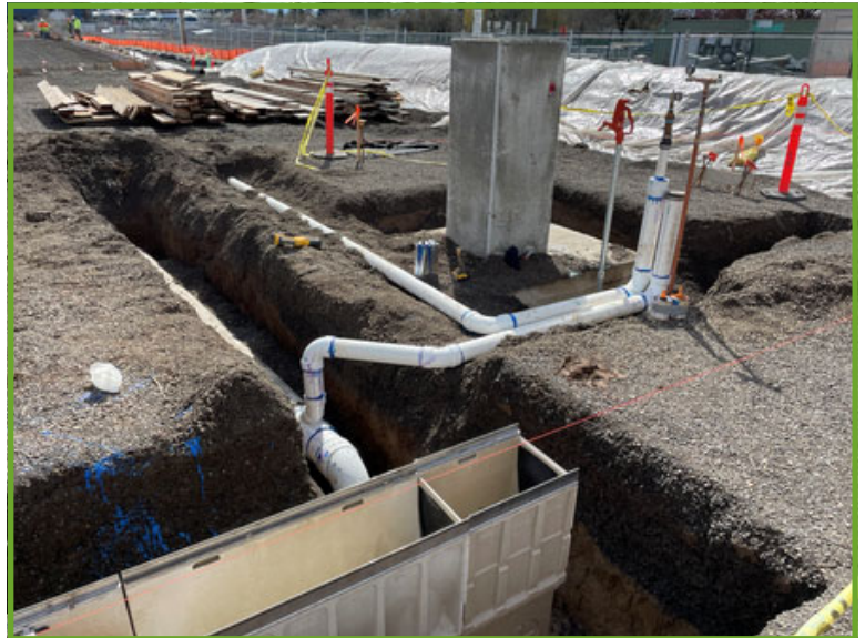
Installation of utilities
