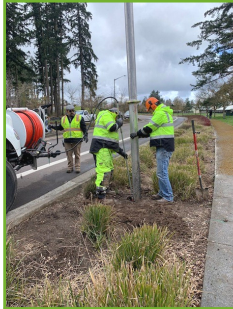
Repairing a line
