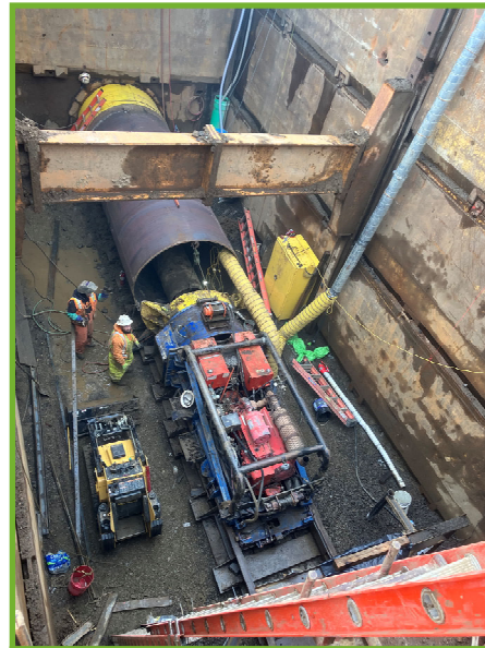
Undercrossing for the WWSP
