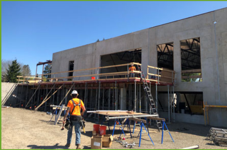
Forming of elevated deck on administration building.
