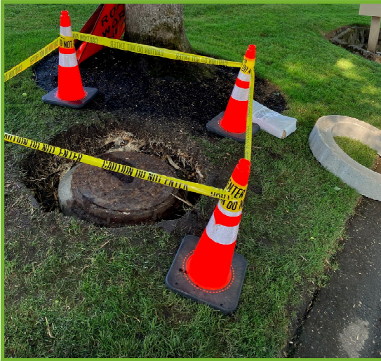
Buried manhole— Before
