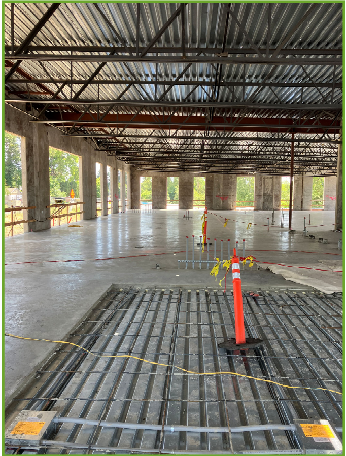
Upper level after concrete flooring was poured—after
