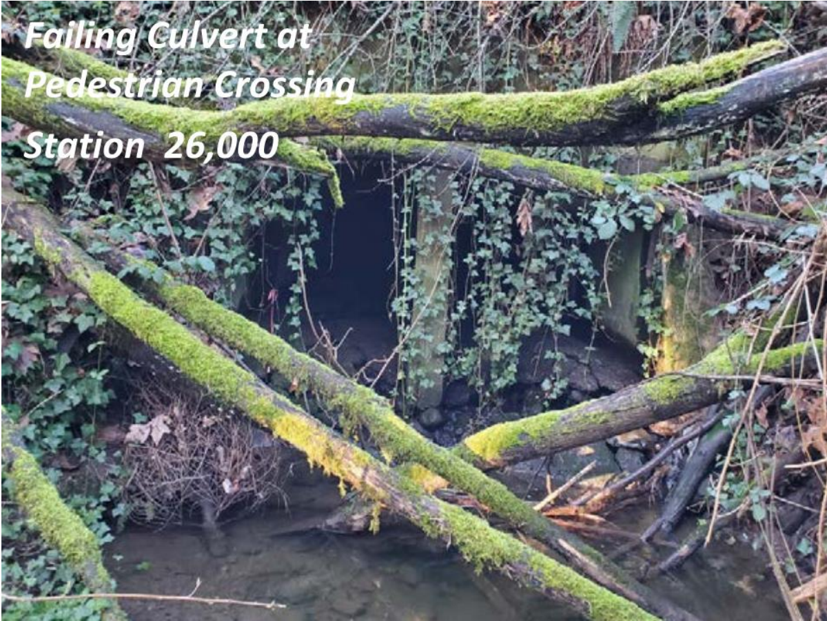
Falling twin 5 ft x 5 ft culverts under pedestrian crossing looking upstream (Source: Geomorphic Stream Assessment, Waterways Consulting, May 2022)
