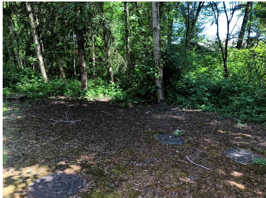
Upstream detention pipes location (May 2023)
