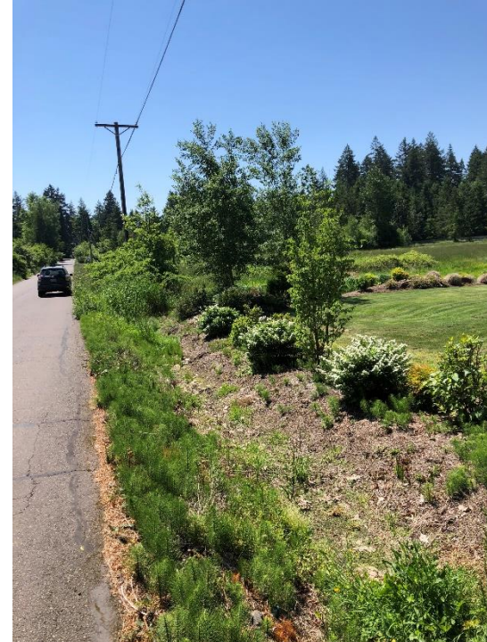
Upstream ditch along west side of Rose Lane (May 2023)
