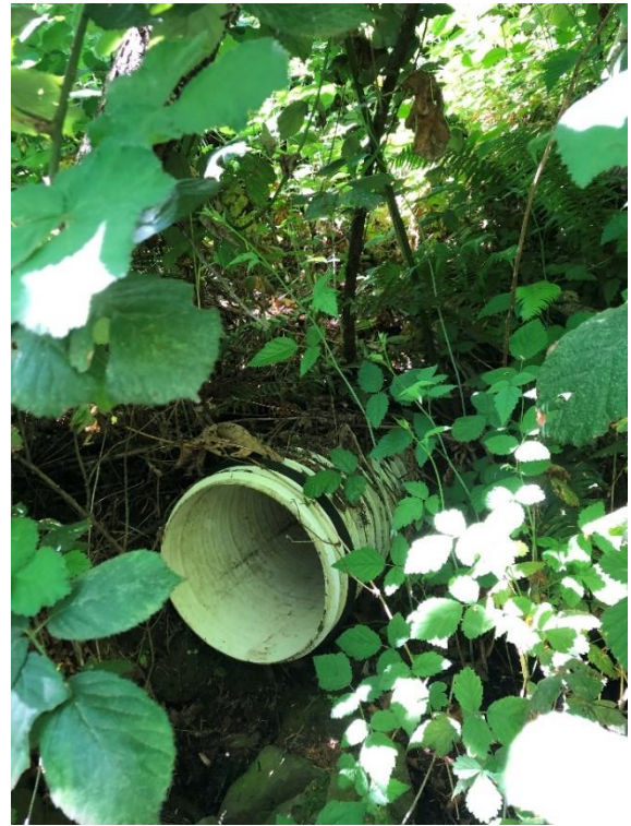
City-owned outfall pipe (May 2023)
