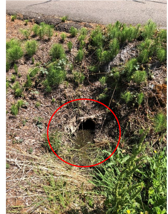
Culvert inlet under Rose Lane (May 2023)
