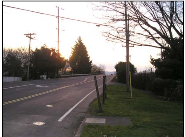
Boeckman Road looking west from Parkway Avenue
