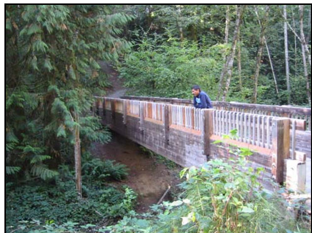
Existing bridge crossing Boeckman Creek
