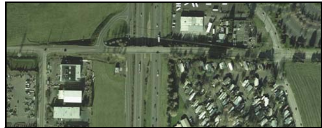
An overhead view of the Boeckman Road overpass
