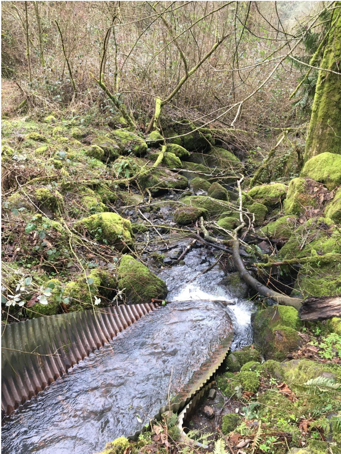
Photo: Boeckman Creek looking downstream from the Boeckman Dip Crossing. The culvert precludes passage upstream from this point, but fish can navigate the rocks at the base of the culvert to reach the crossing.
