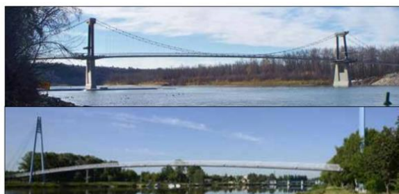
Community members are invited to weigh in with their preference for a suspension bridge (top) or cable stay bridge (bottom). The two bridge types were recommended by the French Prairie Bridge Task Force and City Council for further consideration.
