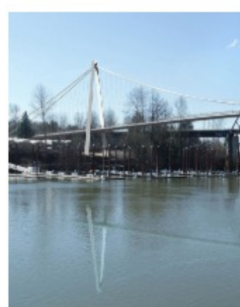
A rendering of the suspension bridge on the south bank of the Willamette River.
