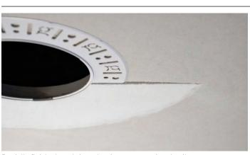
Partially finished mud ring, showing cross-section detail.
