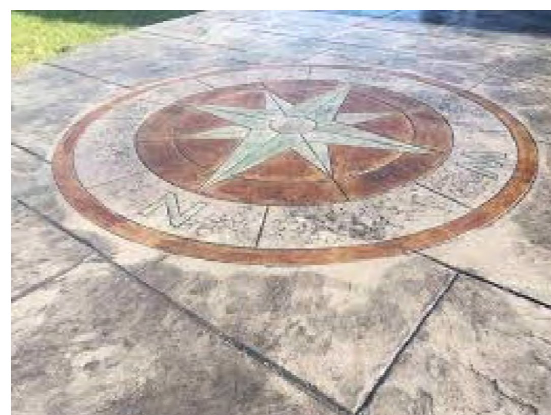
EXAMPLE OF STAMPED CONCRETE SCALE: NTS
