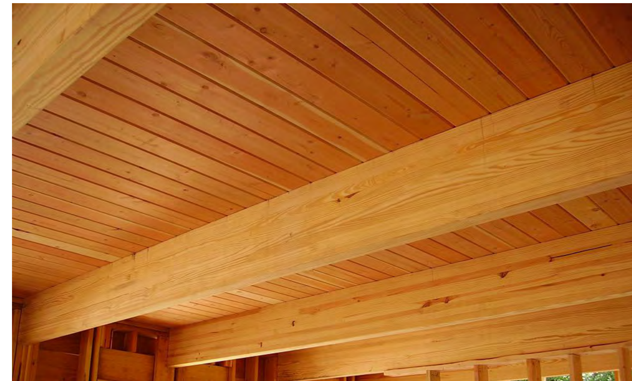
Canopy Structure and Decking
