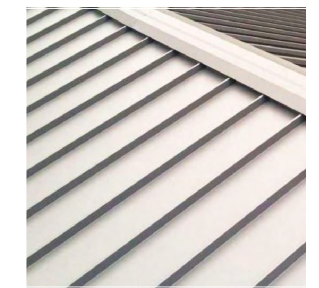
A. Standing Seam Roof Kynar Finish
