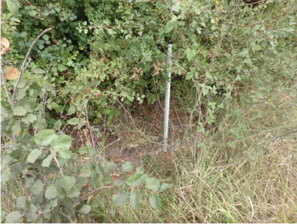
Figure 3. East ditch with left bank 1 ft in height and appearance of overflow path through vegetation. (node 5)
