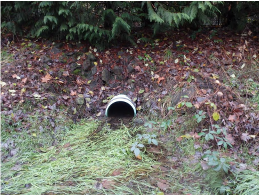
Photo 6 Partly submerged 18-inch CCP contributing culvert
