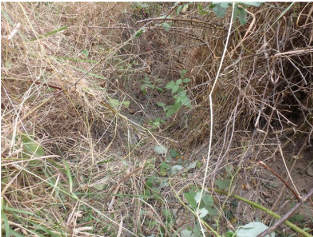
Figure 2. East ditch at outlet of 15" culvert (node 3). Gravelly bottom and heavily vegetated 2:1 side slopes. Roadside right bank 3ft height and left bank 2.5ft height.
