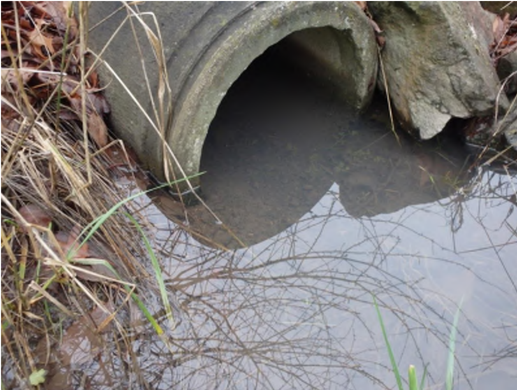
Photo 3 Downstream of culvert with gravel accumulation
