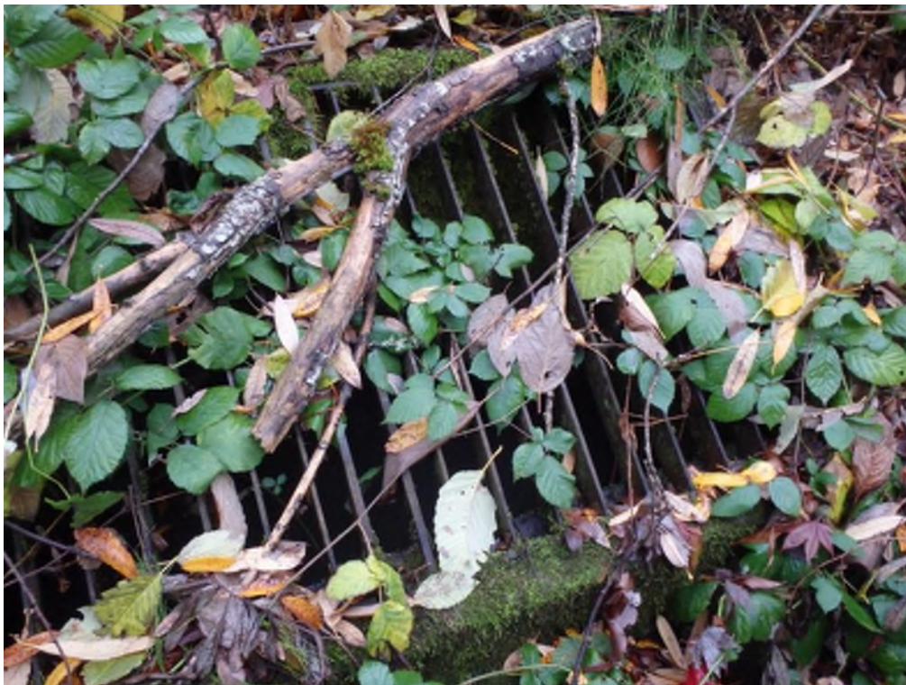
Photo 8 36-inch Outfall into Concrete Box
