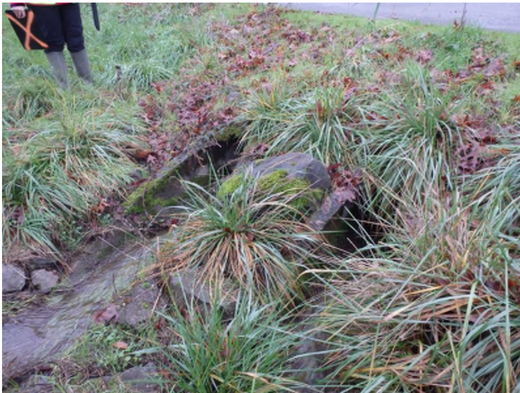
Photo 2 Upstream Ends of Culverts
