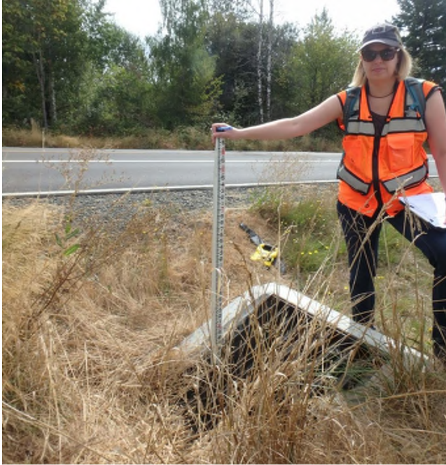
Figure 13. West ditch collected in inlet directly downstream of outfall from church swale. Pipe out to east and connects with discharge from east ditch in manhole and continues south.
