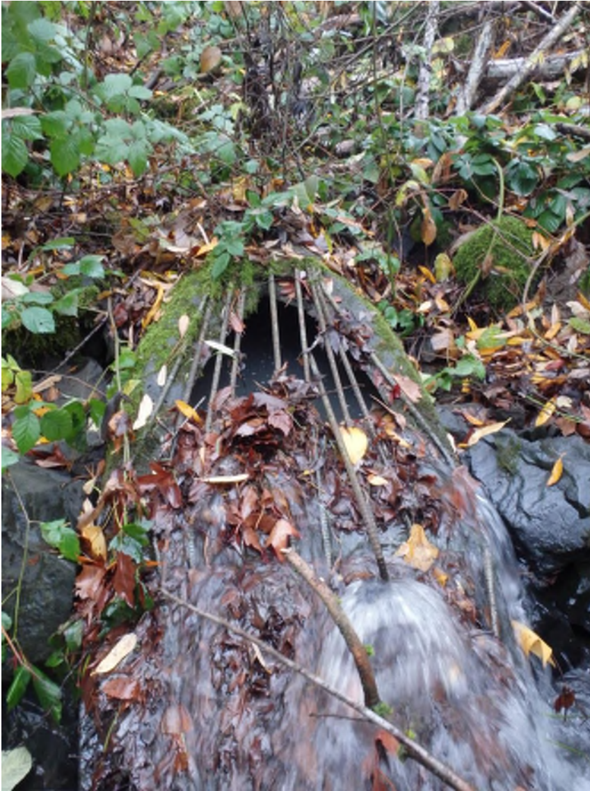
Photo 9 24-inch Outfall from energy dissipation Concrete Box at outfall from 36-inch Pipe
