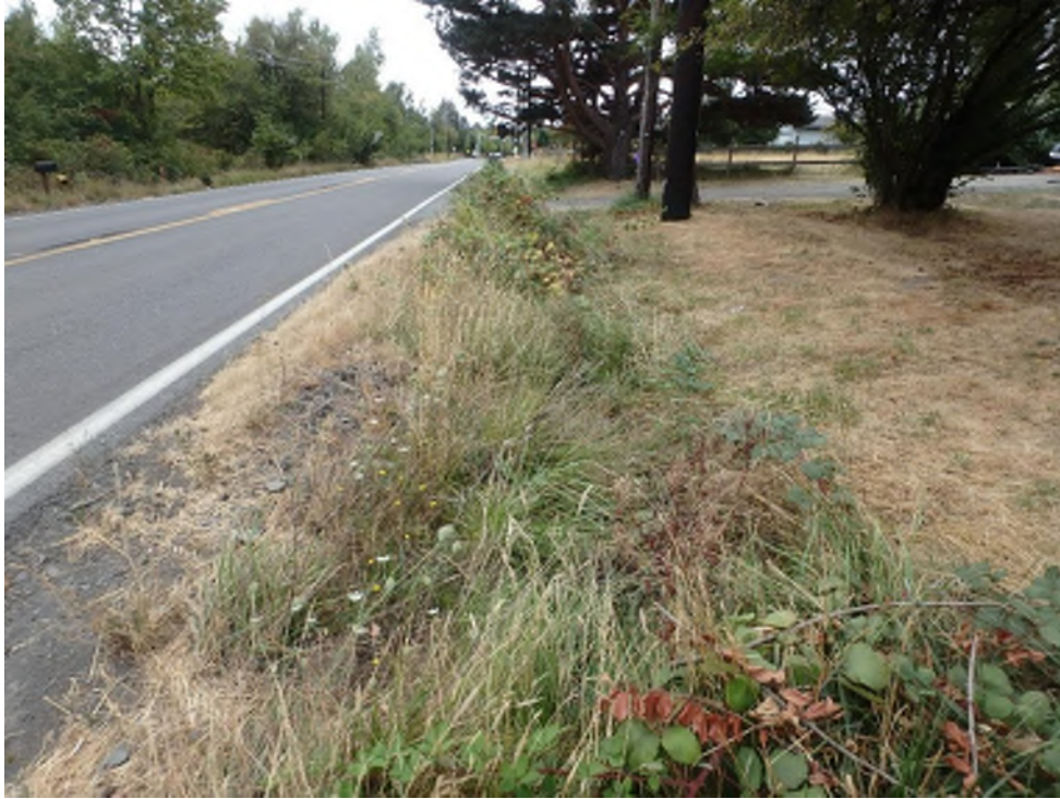
Figure 9. West ditch downstream of 15 inch cross culvert, 2 ft depth, 1.5 ft bottom width and densely vegetated 2:1 side slopes, crosses 4 driveways in 12 inch culverts (Node 21).
