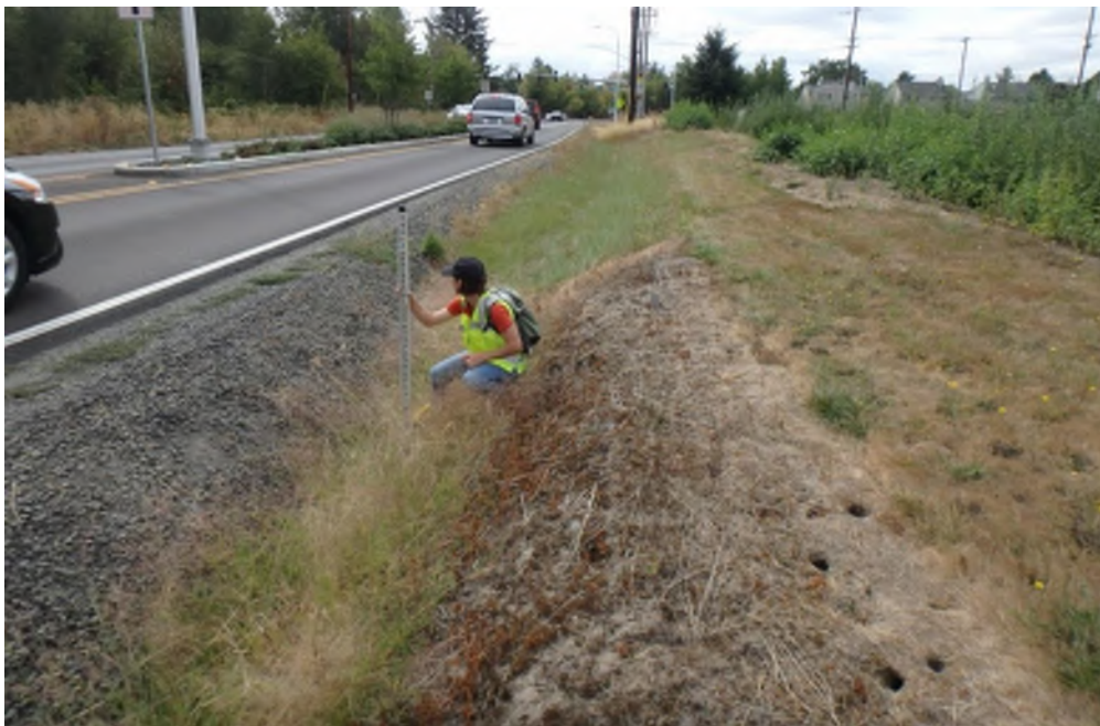
Figure 12. West ditch left bank 2.5 ft high and right bank grassed 3 ft high with transition from 1:1 side slope to 2:1 side slope (Node 31).
