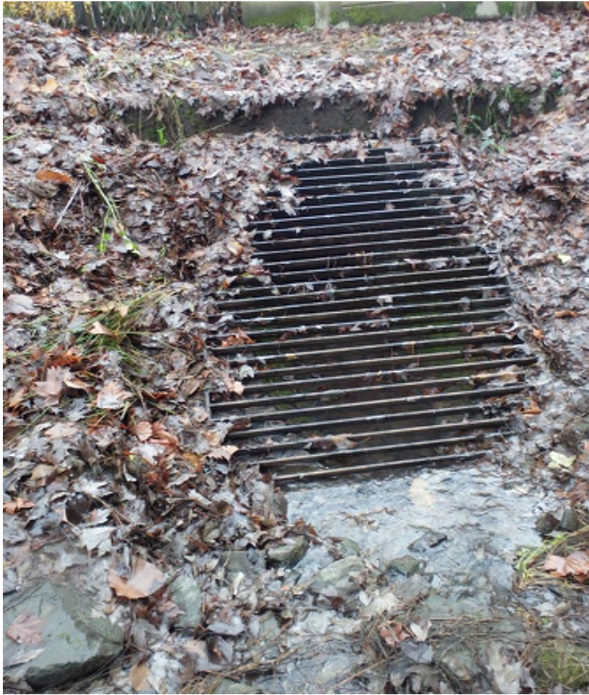
Photo 7 36-inch culvert under SW Willow Creek Drive
