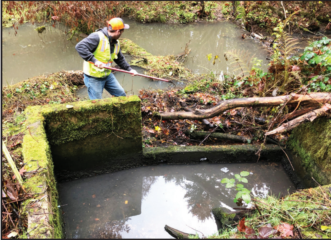
Utilities staff cleaning out a storm outlet.
