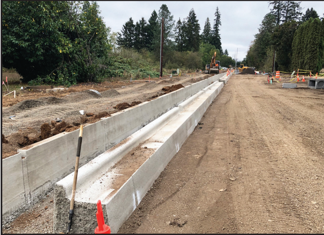
Garden Acres Road under construction during Summer 2020.
