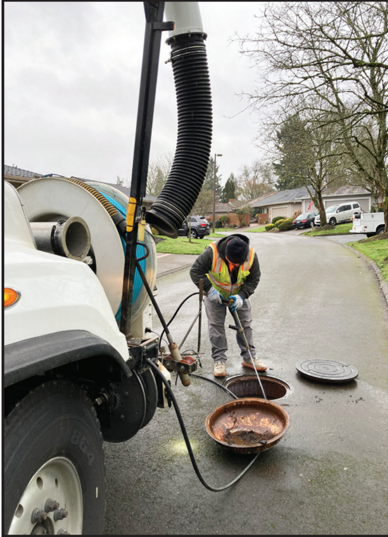
Staff cleaning wastewater lines throughout the City.
