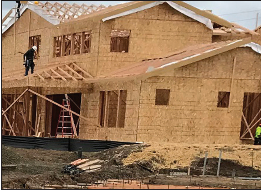
Frog Pond development during construction.
