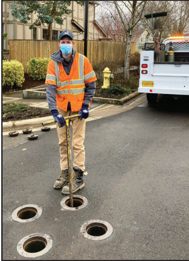
Utilities staff performing maintenance on water valves.
