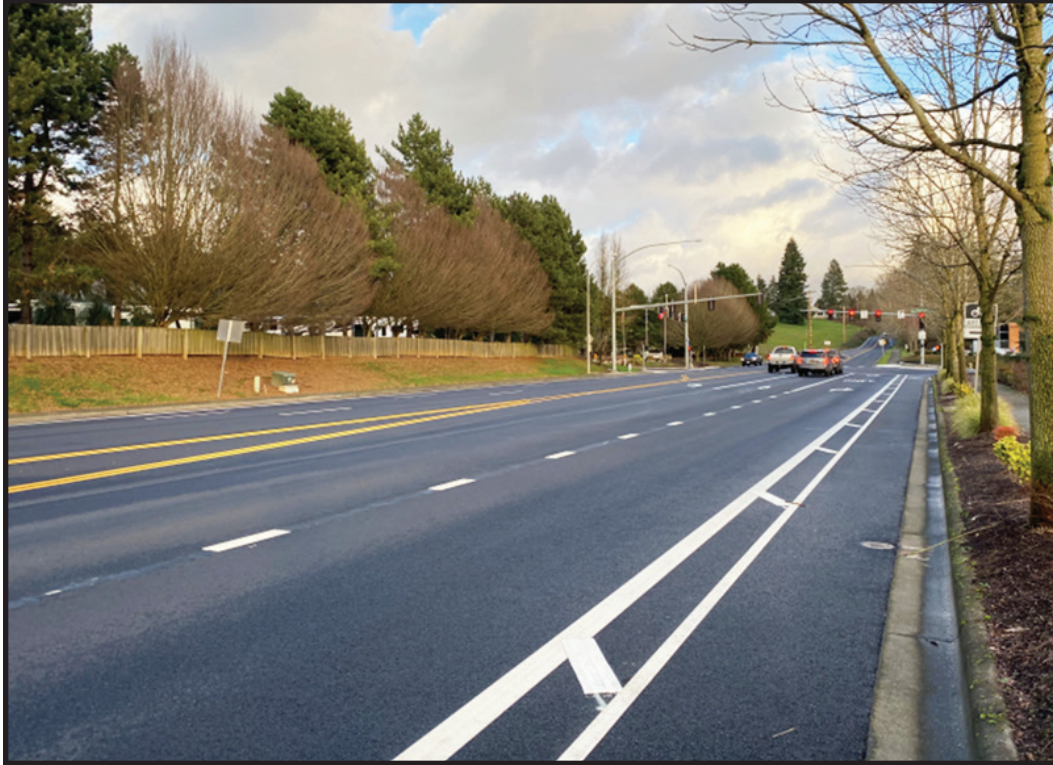
Results of the 2020 street maintenance project.
