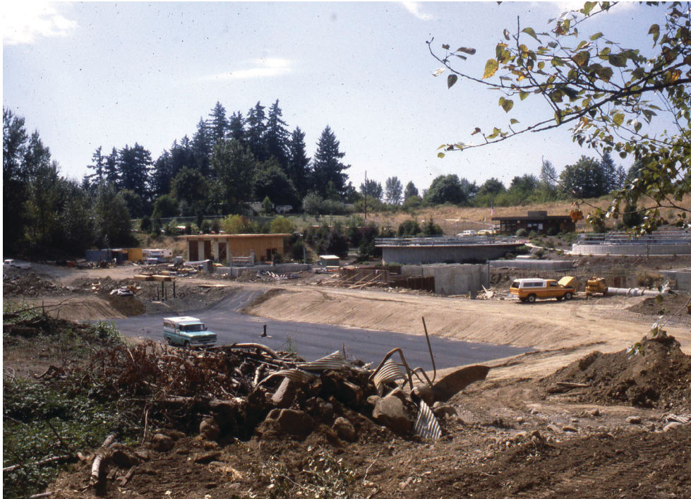
Wilsonville Fred Meyer construction on Boones Ferry Road in 2010
