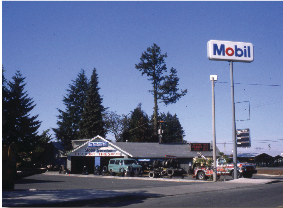
Mobile gas station, formerly known as Bruck's Service Station which was established in 1927 at the intersection known as "Four Corners".
