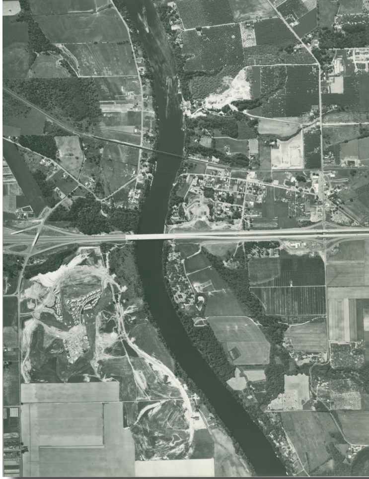
Aerial looking West
