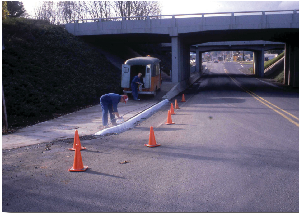
Public Works crew working on Wilsonville Road underpass (circa 1981-1984)
