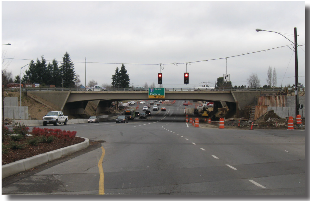
Upgrades being completed to the Wilsonville Road underpass.
