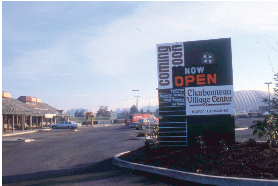
Completion of the Charbonneau Village Center
