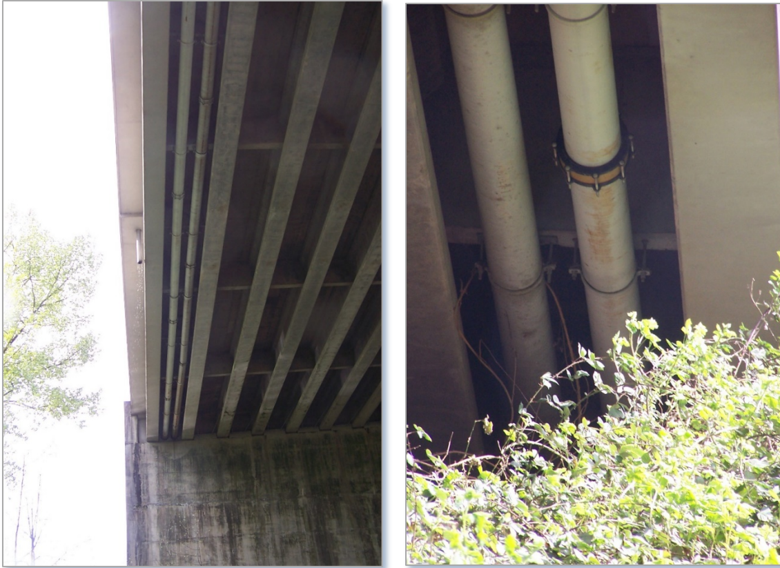
Figure 17: I-5 Bridge River Crossing
