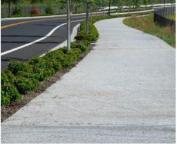
Gaps in the pavers allow water to soak into the ground. Source: Mutual Materials
