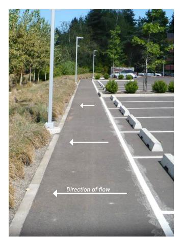
Integrating filter strips with parking areas helps to manage stormwater at the source. Source: City of Wilsonville
