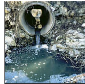
High severity suds Rating: 3 Sewage
