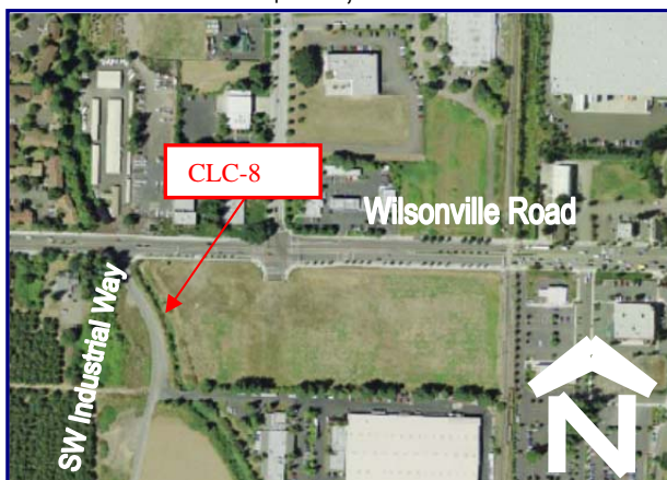
Aerial view of Project CLC-8
