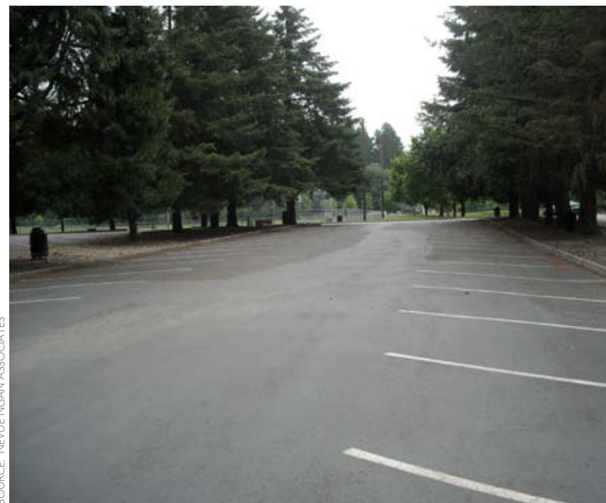
Existing Parking Lot Conditions
