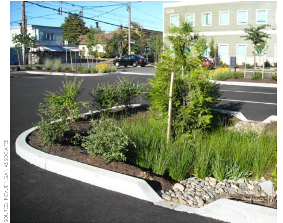
Example: Stormwater Planters
