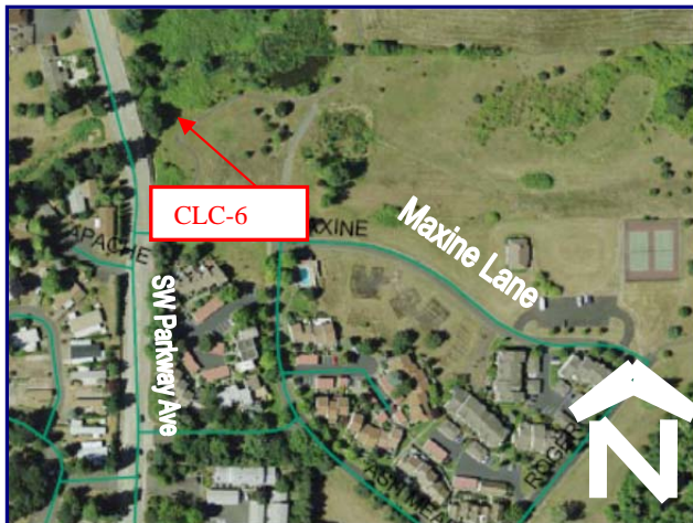
Aerial view of Project CLC-6
