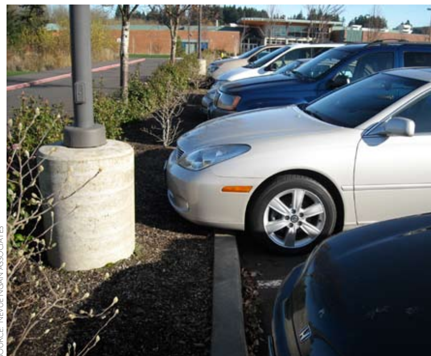
Existing Parking Lot Conditions
