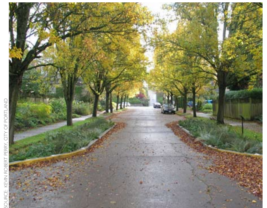
Example: Stormwater Curb Extensions
