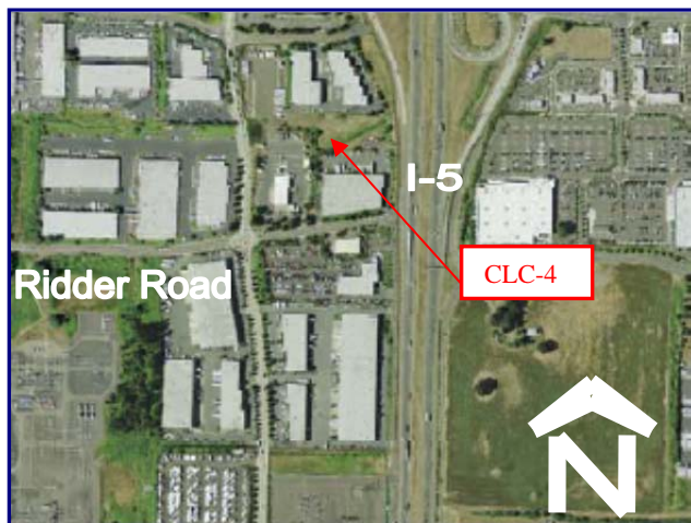
Aerial view of Project CLC-4
