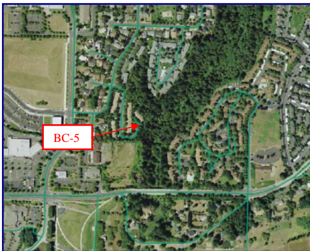
Aerial view of Project BC-5
