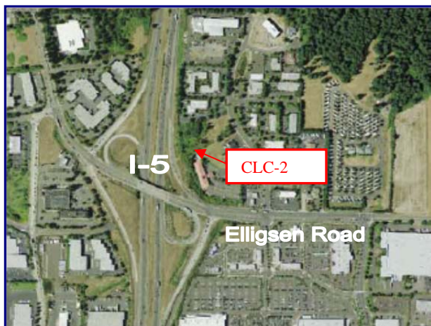
Aerial view of Project CLC-2
