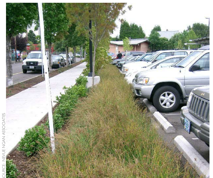
Example: A Green Gutter Within A Parking Lot
