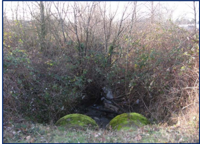
Looking West at Project SD4021 & SD4022
