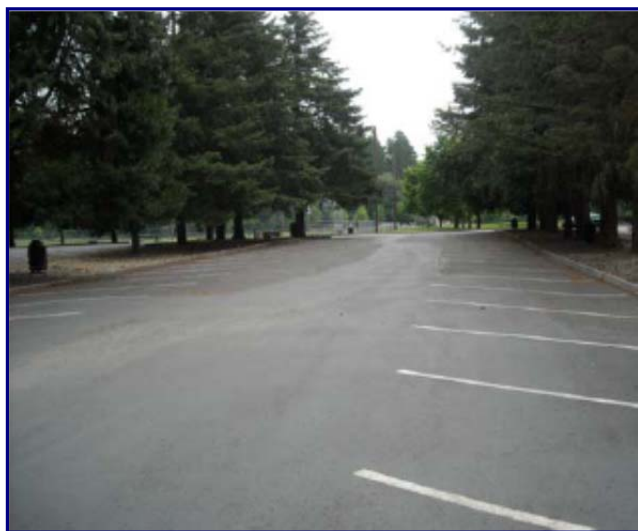
Existing Parking Lot Conditions
