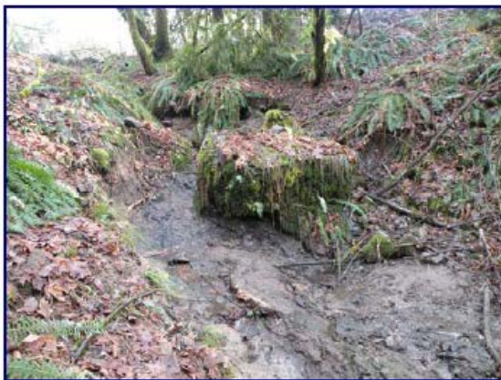
Bank erosion downstream from the Gessellschaft well
