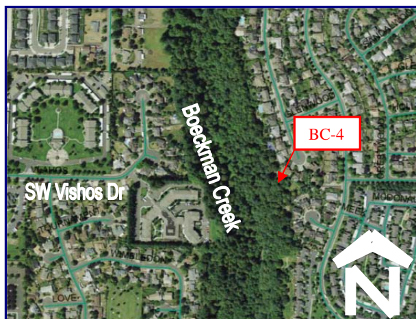
Aerial view of Project BC-4
