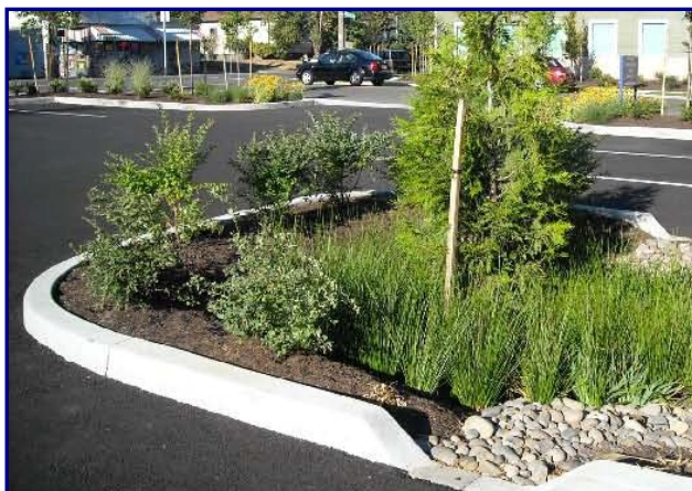
Example of Stormwater Planters in Parking Lot
