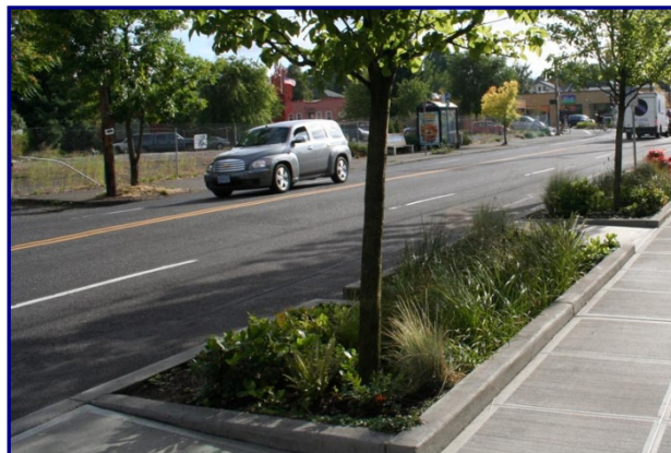
Example of Stormwater Planters with Trees
