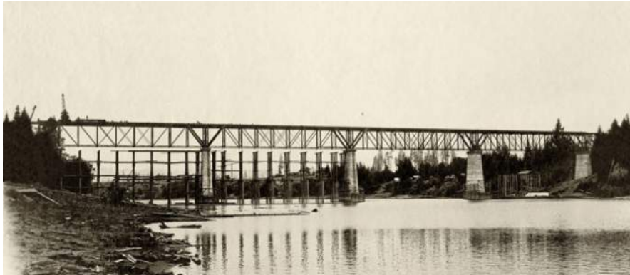
Wilsonville Railroad Bridge Under Construction - circa 1907, Old Oregon Historic Photos
