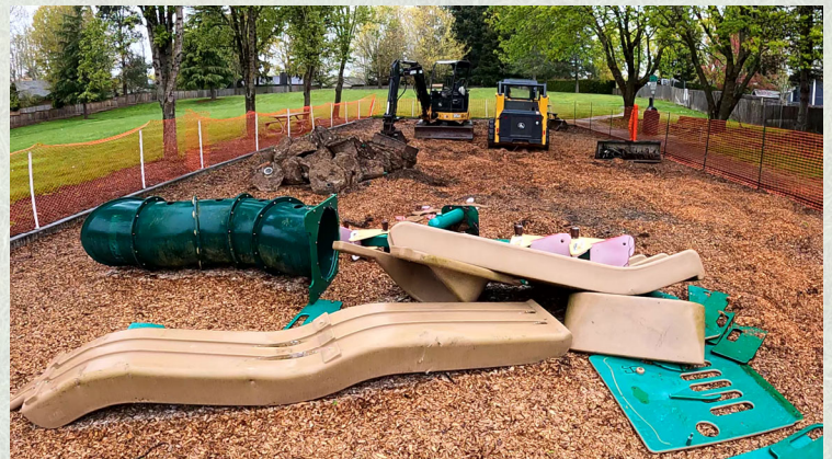
Old Playground Ready for Removal
