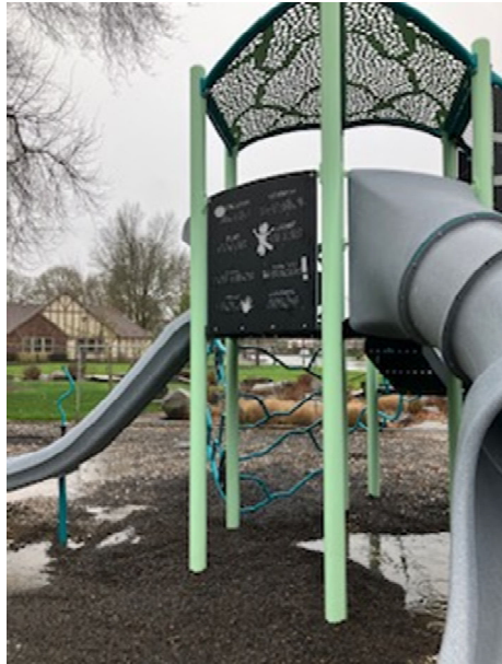
Sofia Nearing Completion
