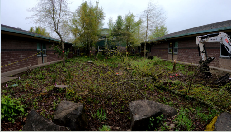
Removal of Material Begins
