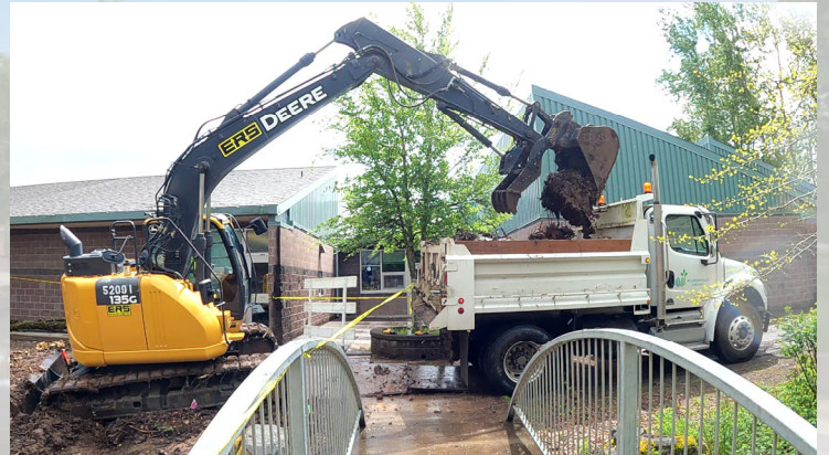
Loading Out Old Fill
