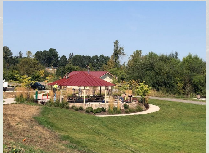
Large Shelter Installation
