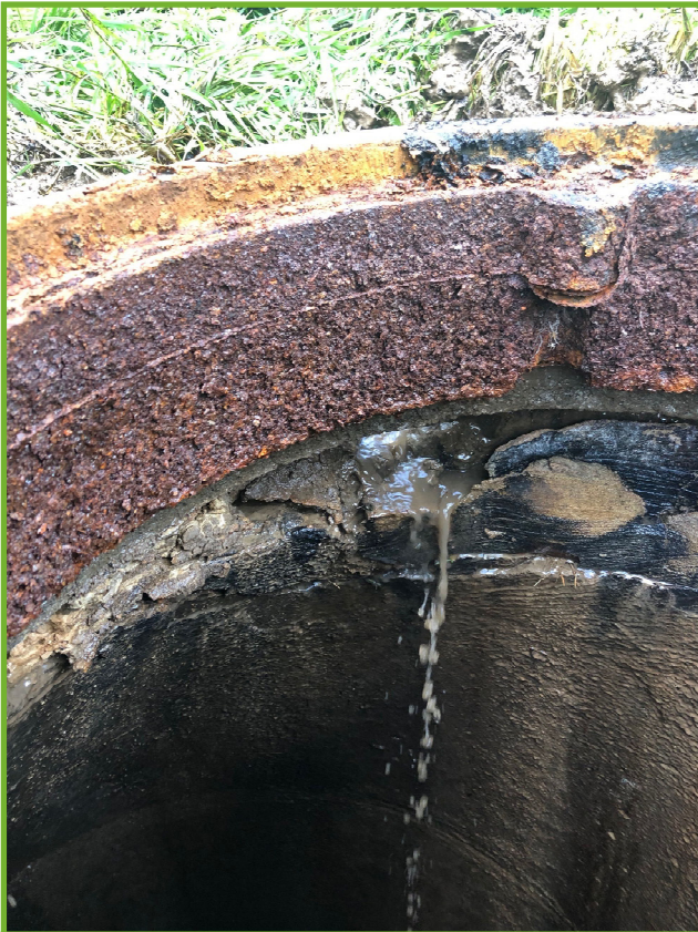
Damaged casting
