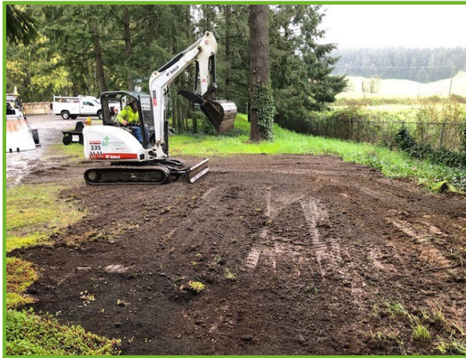
Leveling the site
