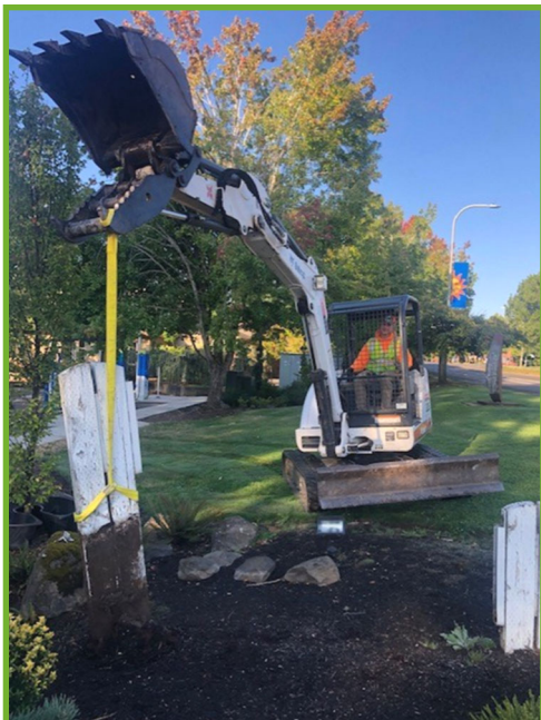
Removing sign posts
