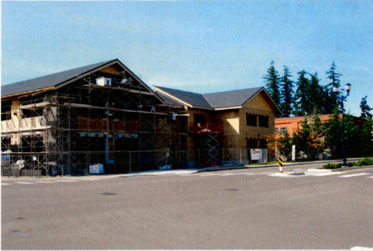
Boone Building near Old Town Square
