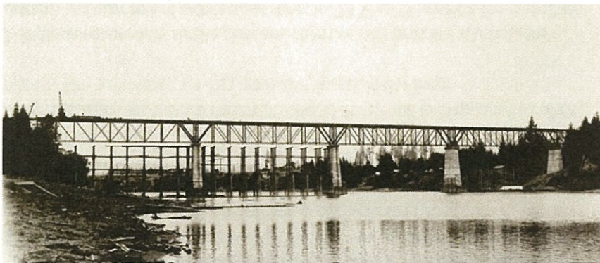
Wilsonville Railroad Bridge Under Construction - circa 1907, Old Oregon Historic Photos
