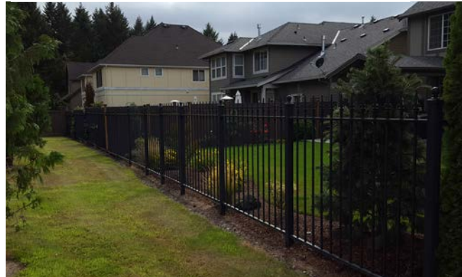
Figure 11. Examples of Creekside Treatment
