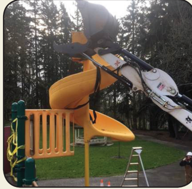
Replaced hazard slide at Boones Ferry Park
