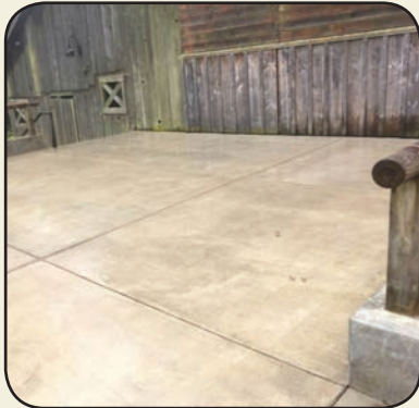
Pressure washed Stein-Boozier Barn in preparation of rental season
