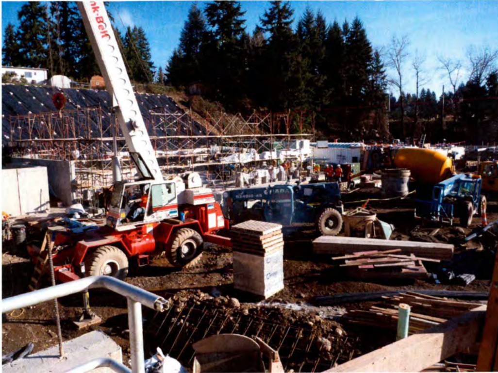
9- Dryer Building masonry construction.
