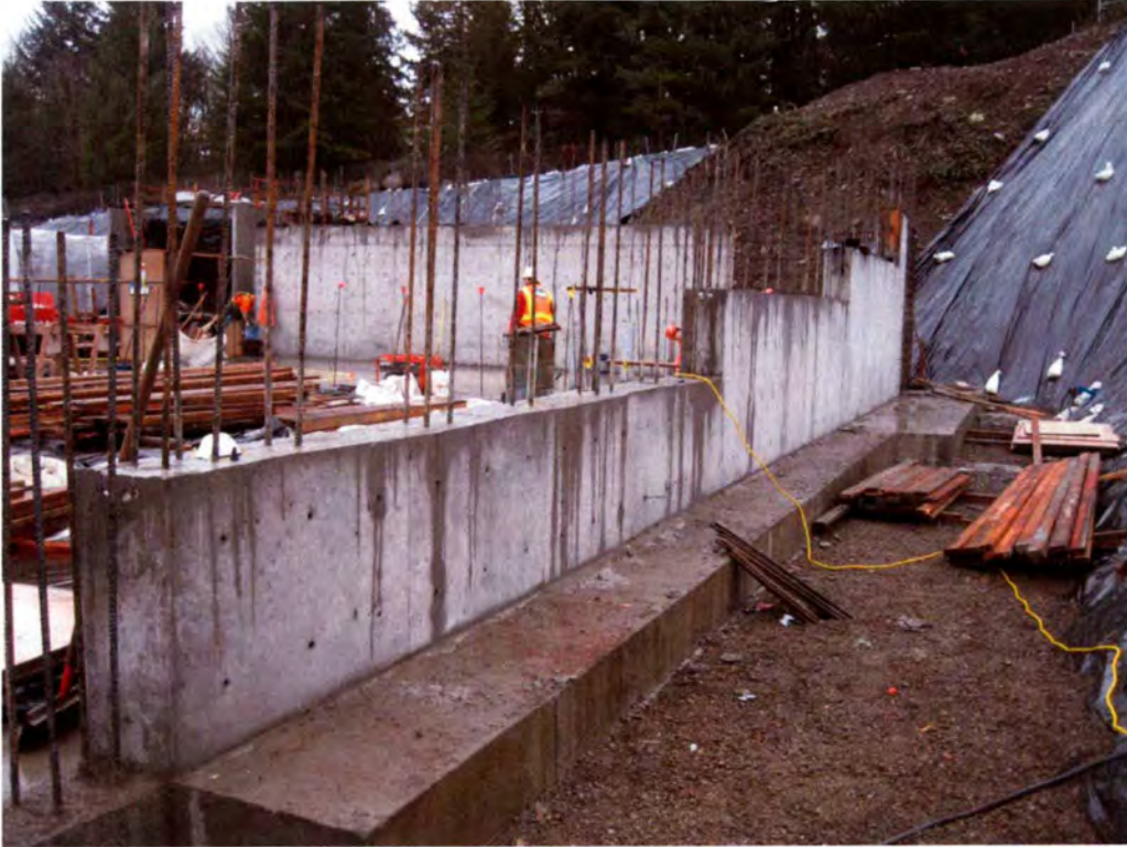
7- North wall at Dewatering and Drying Building.
