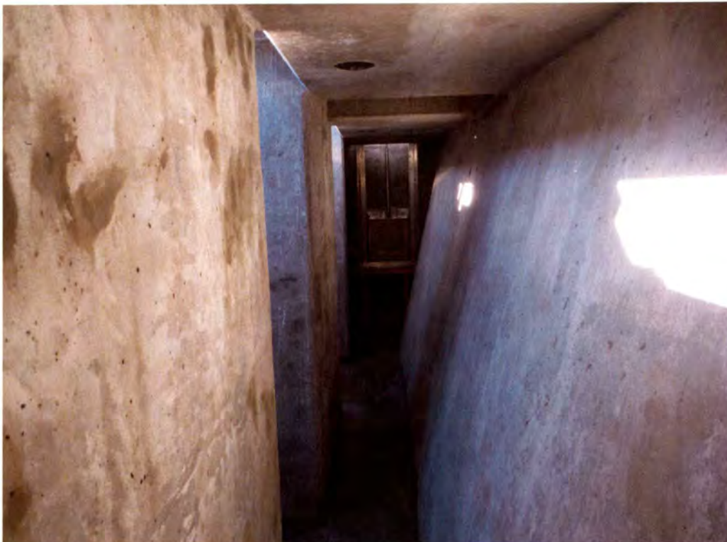
10- Channels in Headworks.
