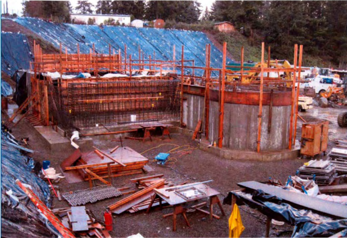
3- Influent channel wall forming.
