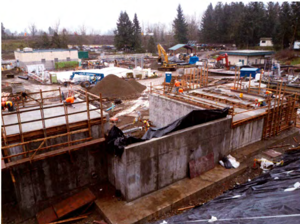
6- Headworks elevated concrete slabs being finished.
