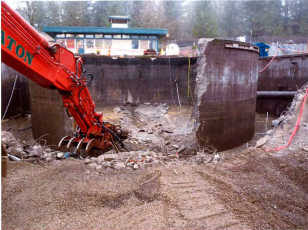
5- Primary clarifier demolition.
