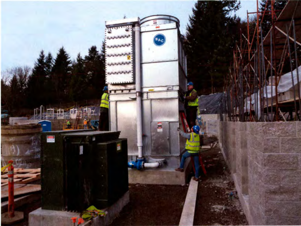
11- Cooling Tower for sludge dryer.
