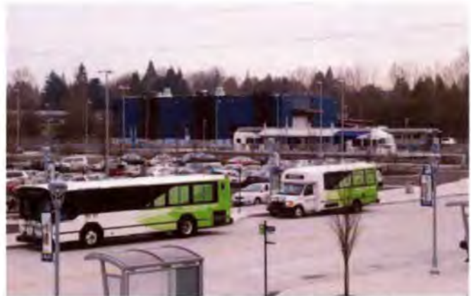
Wilsonville's transit center, SMART Central at Wilsonville Station, is located at the corner of Baber Street and Kinsman Road. It is SMART's main transportation hub and includes a 400-stall park-and-ride lot, twelve bus bays, an operator break room, public restrooms, shelters, and a clock tower with security cameras. It also shares the site with TriMet's Westside Express Service (WES) commuter rail station. Wilsonville is WES's southern terminus.
