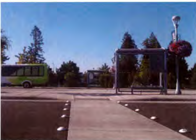
Curb ramps with gradual slopes and large transit pads at the SMART Central transit center can accommodate users in wheel chairs or with other special needs.
