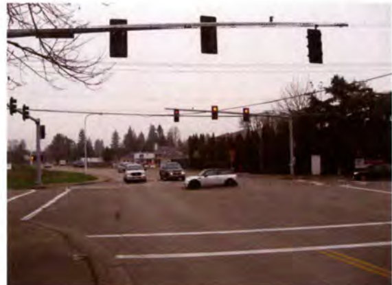
The Parkway Ave. Boeckman Rd. Traffic Signal Improvements
