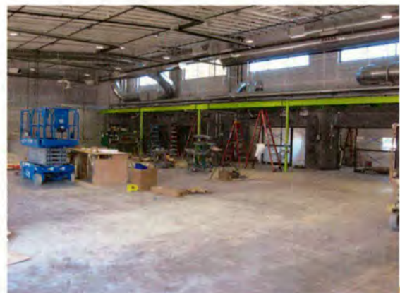
SMART Ops/Fleet Maintenance Building
