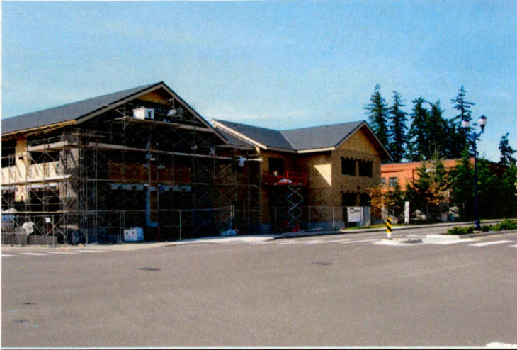
Boone Building near Old Town Square
