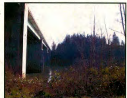
West side of I-5 bridge
