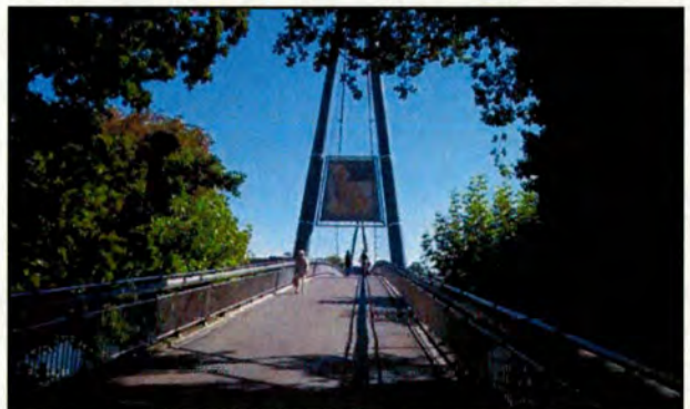
Bicycle/pedestrian suspension bridge in Frankfurt, Germany
