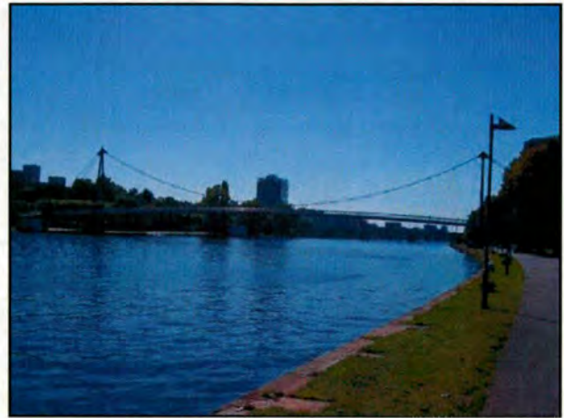
Bicycle/pedestrian suspension bridge in Frankfurt, Germany
