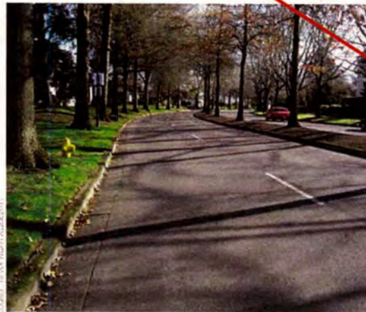
Existing Parking Lot Conditions
