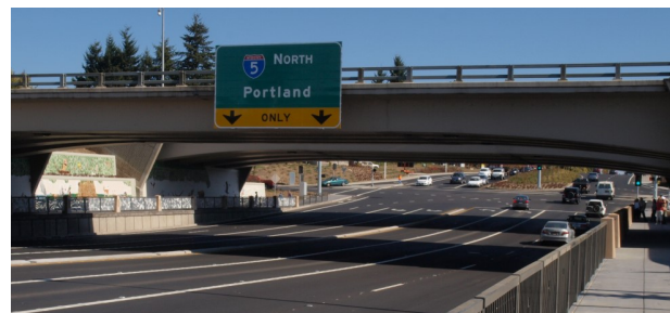
Looking east to the I-5/Wilsonville Road interchange.
