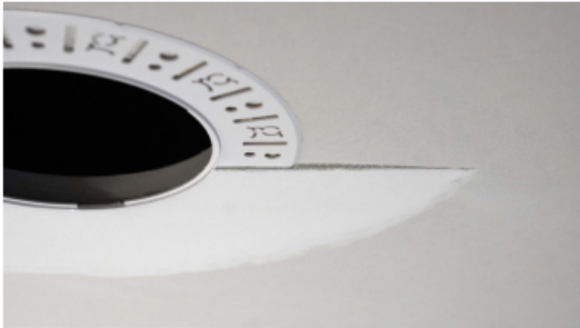
Partially finished mud ring, showing cross-section detail.
