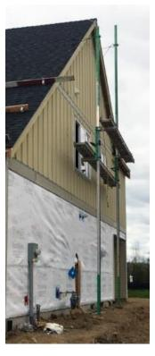
I believe the only vertical pole / scaffold system that was used (mounts into shingle area of roof) was that installed and used by the Siding contractor. This picture is an example of such a system from a home at Frog Pond.
