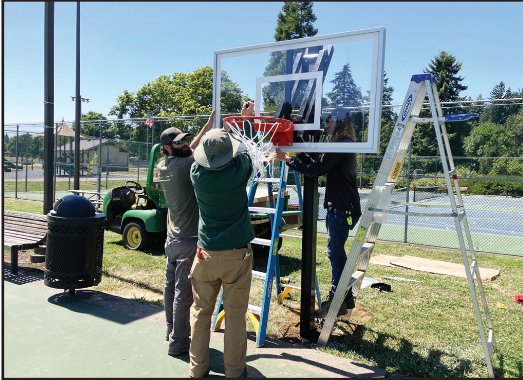
Park Maintenance staff replacing a basketball hoop.
