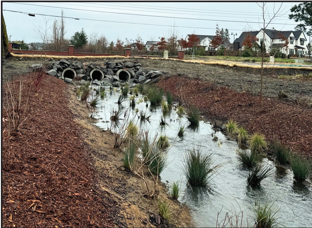
Meridian Creek culvert upsizing and stream restoration completion (CIP #7067).
