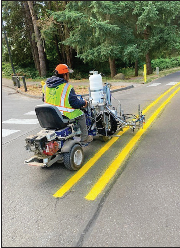
Roads staff applying centerline striping to Memorial Drive.
