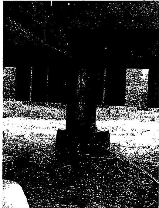
FOUNDATIONS AND FLOOR FRAMING *Wood and stone foundations with hand-hewn floor framing timbers.*
