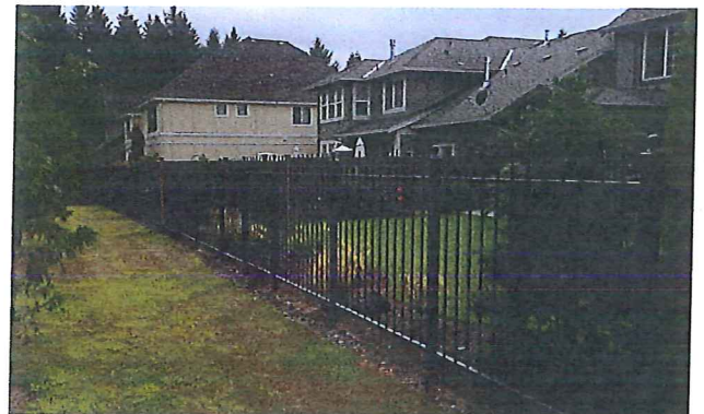
Figure 12. Examples of Creekside Treatment
