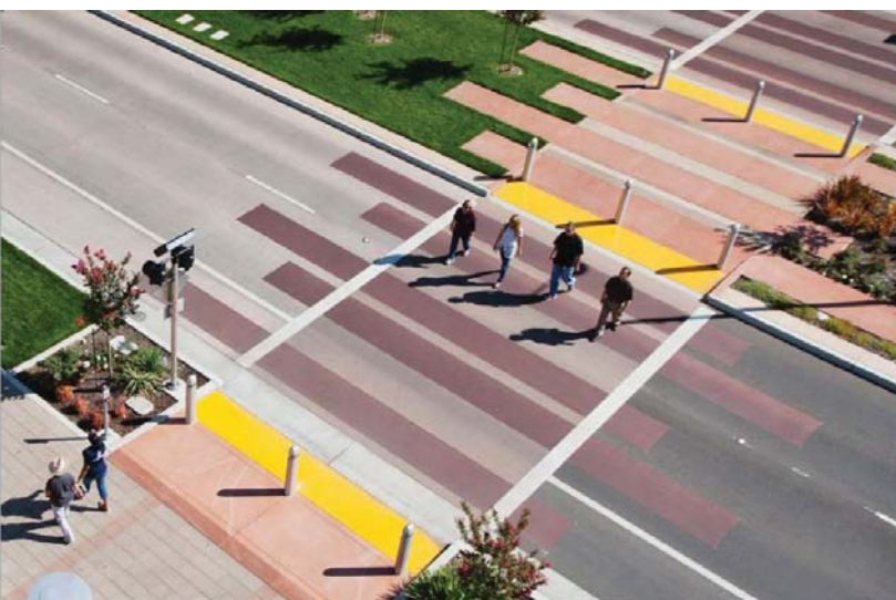
highly visible pedestrian crossing
